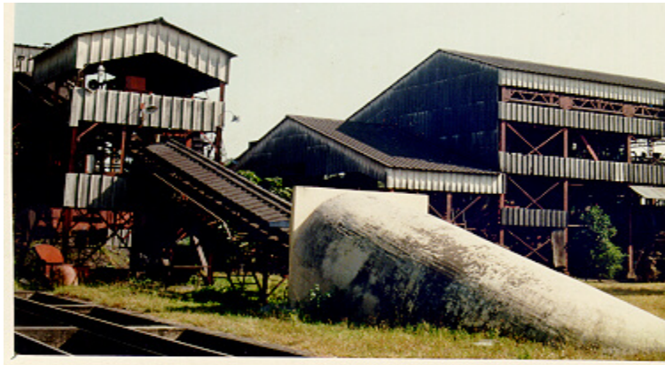
Coal Washing Pilot Plant
